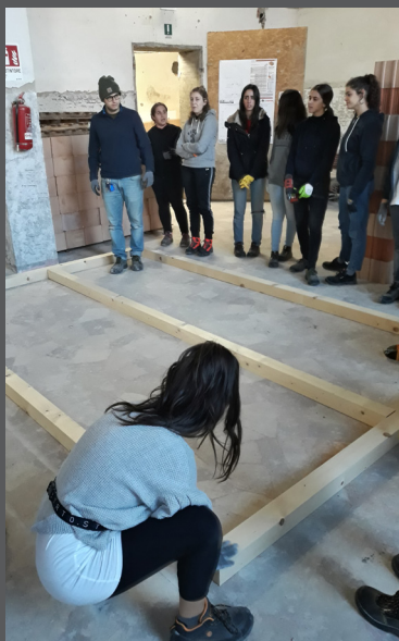
New metering box construction
